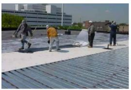
USG Securock Over Metal Deck Substrate
